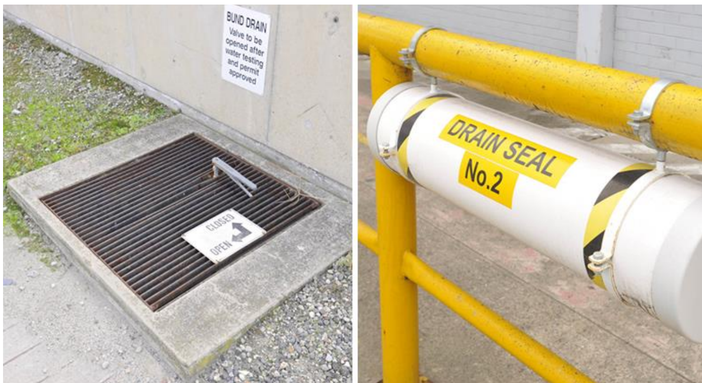
Figure 15: Site isolation systems can be used to cut off a site from the stormwater system during an incident such as a spill or fire at times of high risk.
