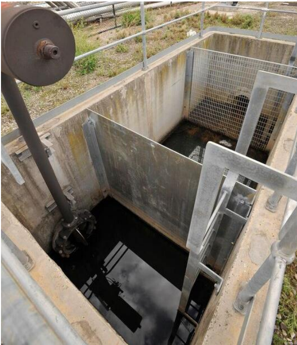
Figure 3: Image of a triple interceptor system. This system will retain contaminants such as oil, grease, sand, silt etc. as water flows through the three tanks. This will prevent the pollutants from entering the stormwater system.
