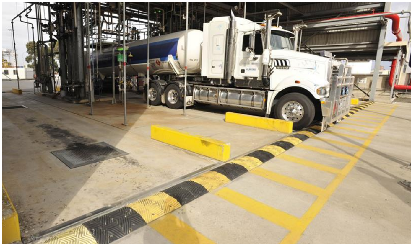
Figure 14: Rollover bunds can be a useful form of containment that can prevent liquids from leaving the work area.
